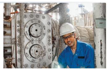
Believing output for its two LLDPE lines was gearpump limited, EQUATE replaced old units with two Maag PR 32 pumps and experienced a whopping 39% increase in throughput, says Mohammad Al-Qahtani, EQUATE's senior technical advisor for polyethylene.
